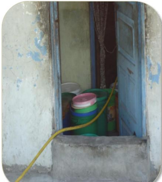
Figure 2: Other private people have connected Pipes connected from water sources for supplying water in households
