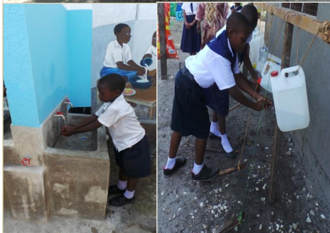
Pupils washing hands at the installed hand washing facilities
