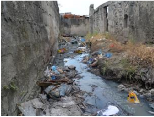
Mzinga drainage channel, Pakacha
