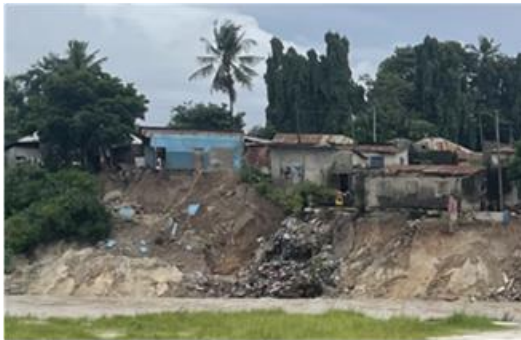
Erosion of Msimbazi riverbank, Kombo
