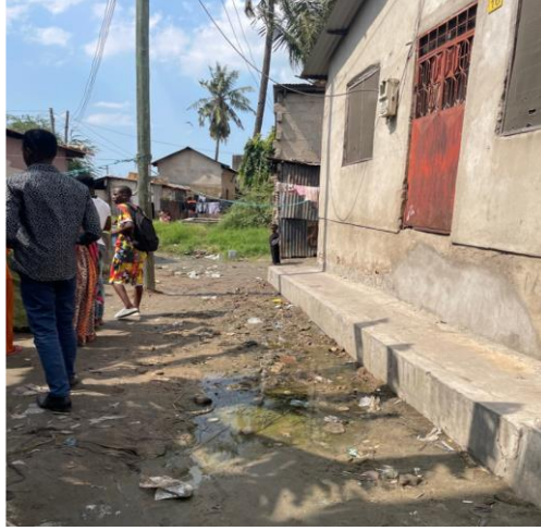
Raised doorways to avoid flood, Pakacha
