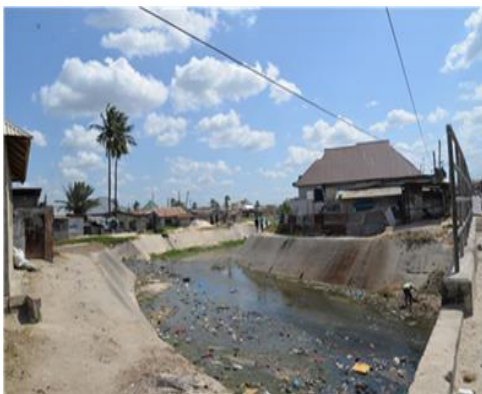
Improved Ng'ombe River embankment, Tandale
